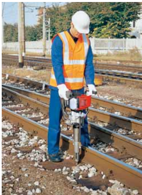
FIG. 5 USING THE DRILLING MACHINE INDEPENDENTLY
